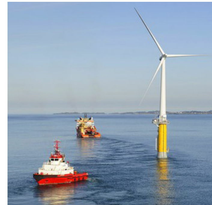
Hywind turbine being towed at sea in deep water
